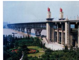
1st Yangtze Bridge: 1968
